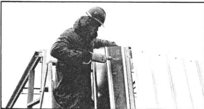
SWCN Russel Laurel drills holes for securing building wall.
