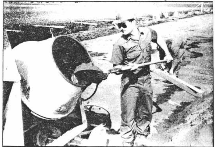
EO3 Scott Grignon adds sand to the concrete mixer.
