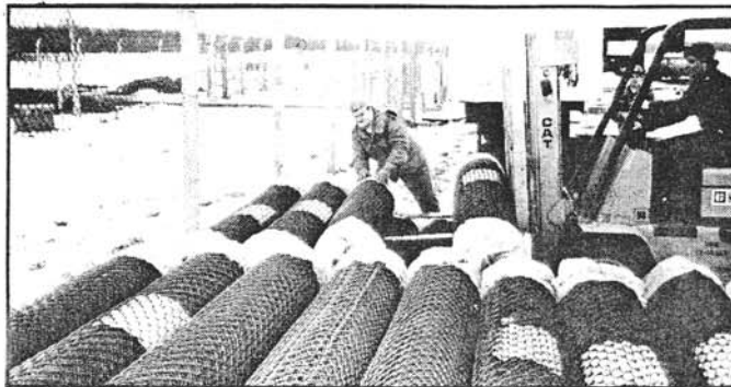
BU2 Bob Tunstill off-loading fence fabric for the new Ops Area security perimeter.
